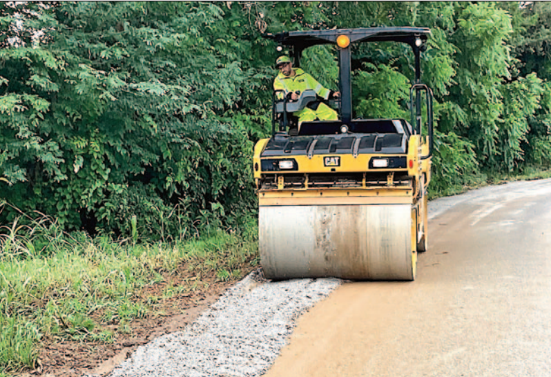
Kentucky Transportation Cabinet crews were busy last week building shoulders on Tabor Road in rural Crittenden County because it's getting an unusual amount of traffic due to a bridge out on KY 295 between Dycusburg and Eddyville. The narrow country road is one of the shortest detours around the closed bridge. The bridge, which spans Livingston Creek on KY 295, will likely be closed through the rest of 2024.
